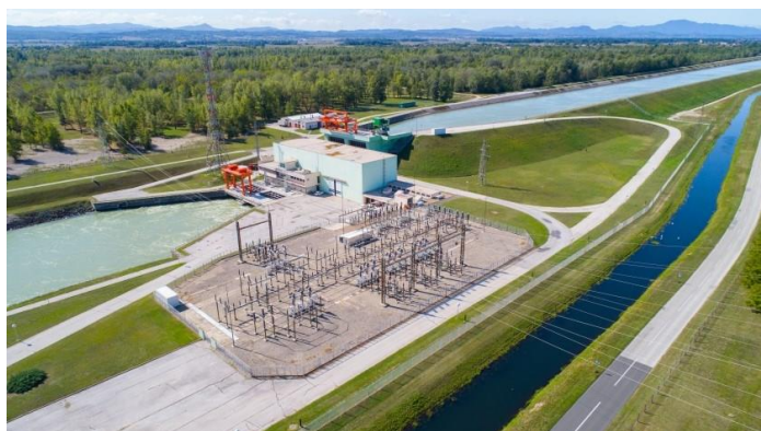
Figure: Hydroelectric power plant Čakovec (Source: Hrvatska elektroprivreda HEP )
