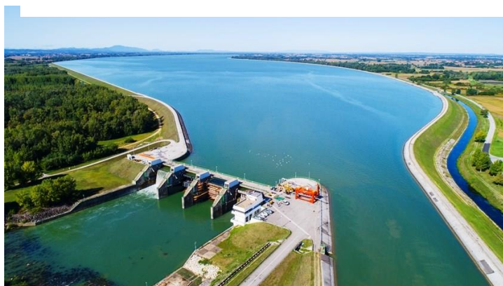
Figure: Hydroelectric power plan Dubrava (Source: Hrvatska elektroprivreda HEP )
